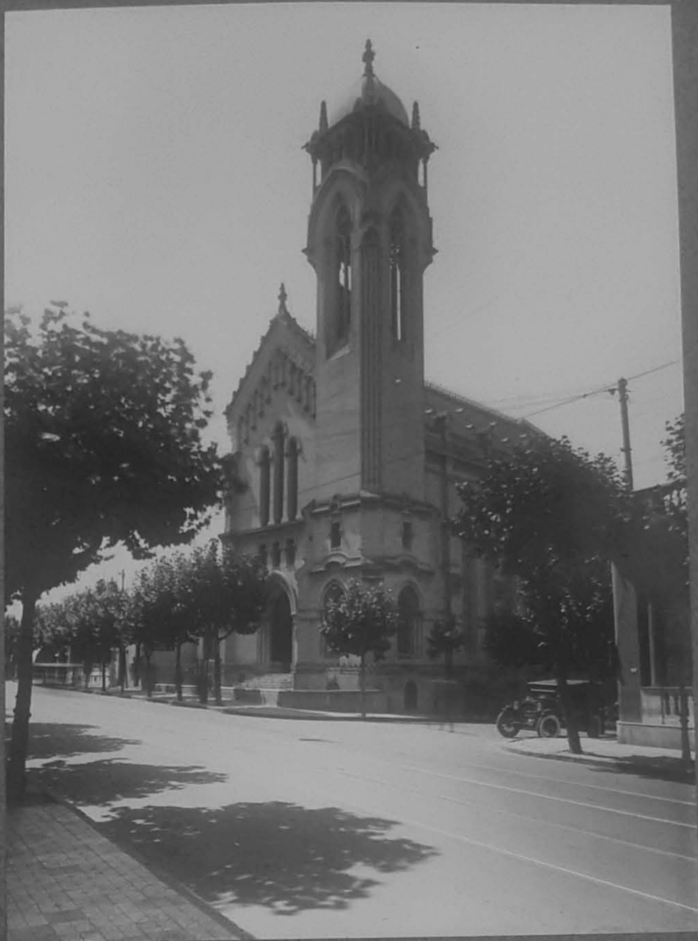
Central Church - McCabe Memorial Hall on the ground floor.
