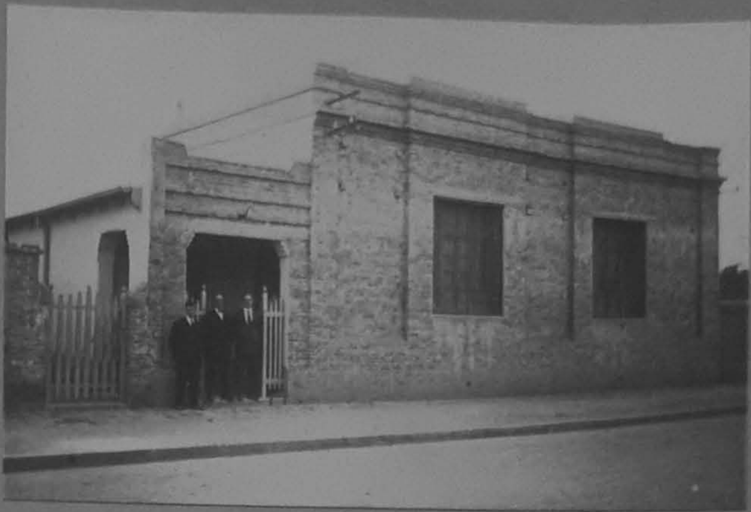
Hall and school building - Arrogito, Rosario. -
